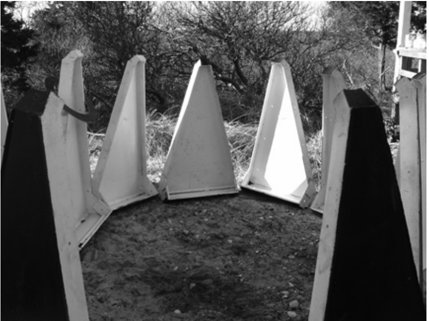
The cast iron roof pieces for the new lantern room. Painted black on the outside and white on the inside.
