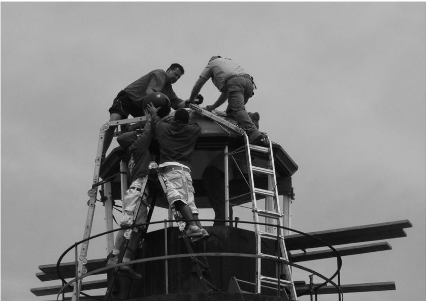
Almost there - installation of the vent ball
