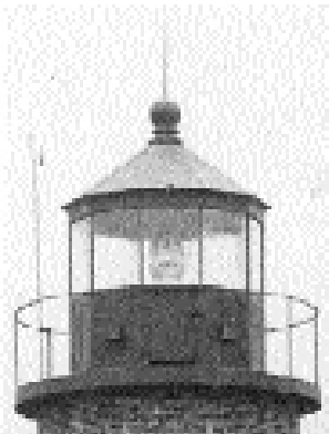
(left) Close-up of the lantern house with Fresnel lens visible.
