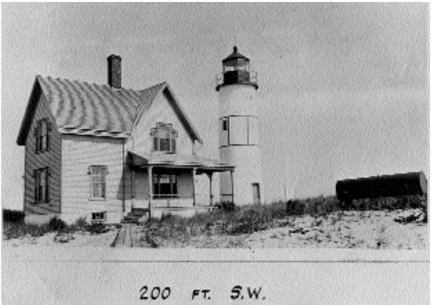
Photo: “200 FT. S. W.” 1930 or ‘31. [4 - 26] Just before decommissioning/darkening of the tower. Note the absence of the entrance room and the wood house and the presence of the oil tank, for the new incandescent oil vapor light source.
