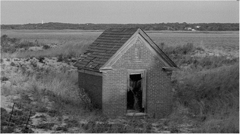
Oil House, built in 1905. Summer, 2004. [4 - 21]
