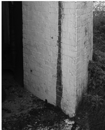
(below right) Entryway to tower showing thickness of tower wall - 3 feet - at the base. (Door has been removed for restoration)
