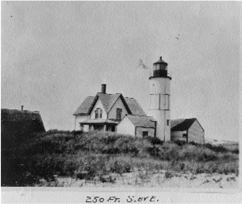
Photo: "250 FT. S. BY E." c.1920. [4 - 25]
