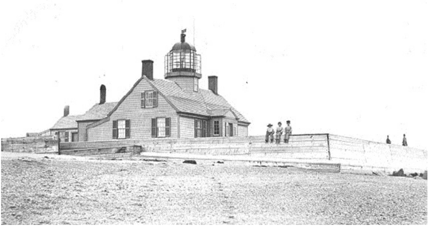
The original Long Point Lighthouse, built 1827 in Provincetown. This photo and the next illustrate the unified house and tower design of the first Sandy Neck lightstation. [3 - 1]
