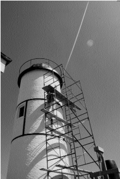
Scaffolding for repainting the tower.
